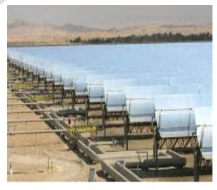
Solar paraboloids use a Parabolic Trough Collector system, which includes long, curved mirrors designed to concentrate sunlight onto a receiver tube located at the mirror's focal line.
